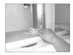
16. Connect duct to opening, inspect and tape all joints with approved aluminum or duct tape.
